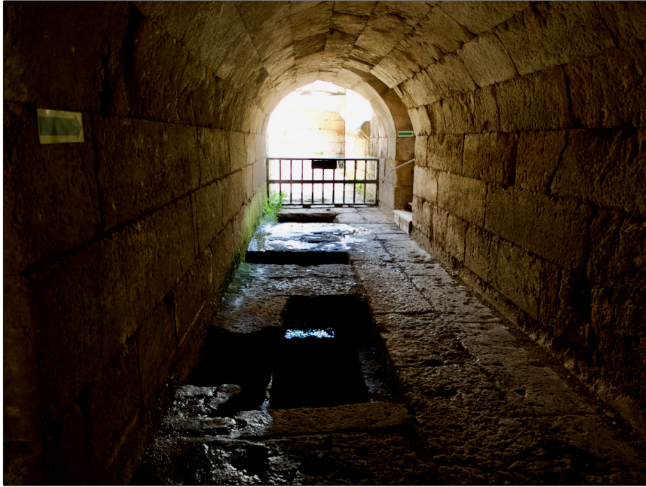
Tunnels under the Palace of Herod Agrippa II (May 2022)
